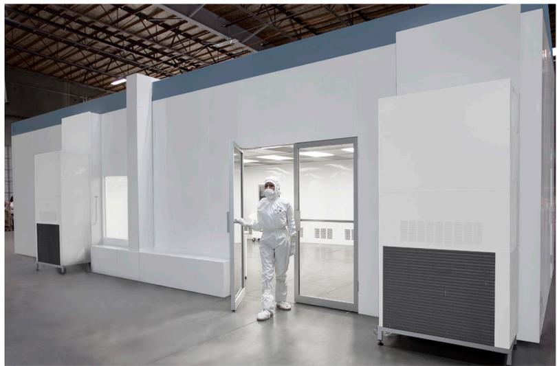
Negative-pressure containment BioSafe® cleanroom, showing return ducts to ceiling-mounted exhaust fans.
