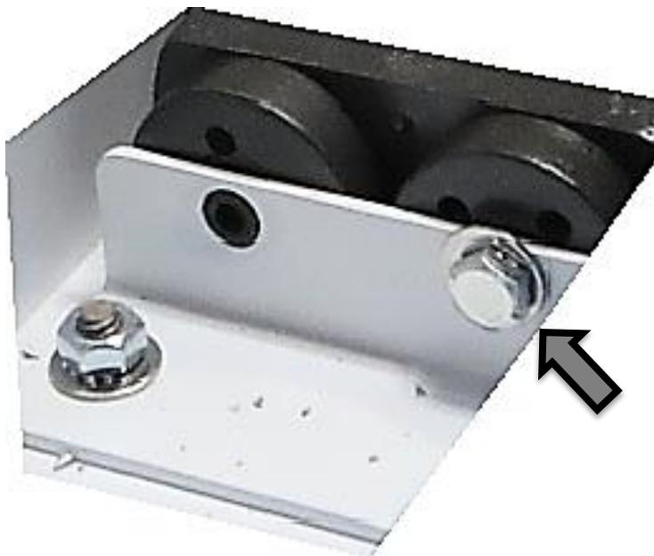
Figure 13: Screw that needs to be adjusted on concealed door closer to fix tension
