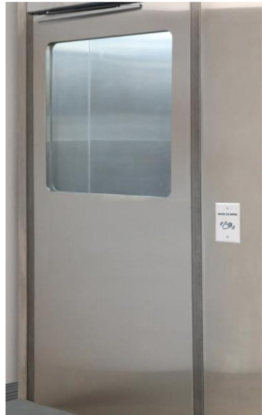
Figure 10: Stainless steel door with partial view tempered glass window and automatic opening sensor
