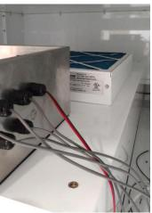
**Figure 7.** The blue MERV 7 pre-filter can be lifted out and replaced with a new one
