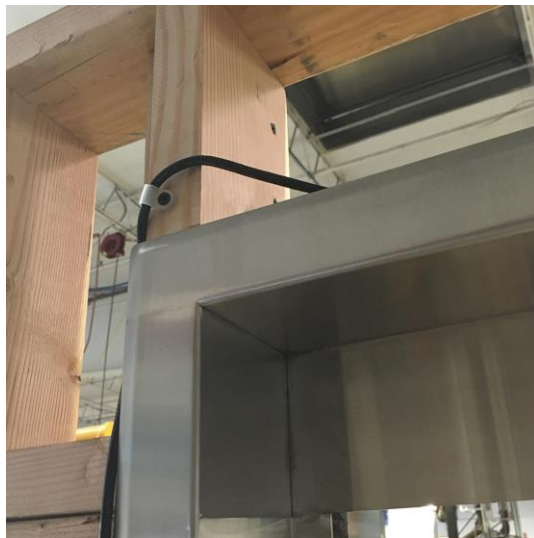
Figure 2: The “Clean side” of the door frame features a smooth, tapered edge
