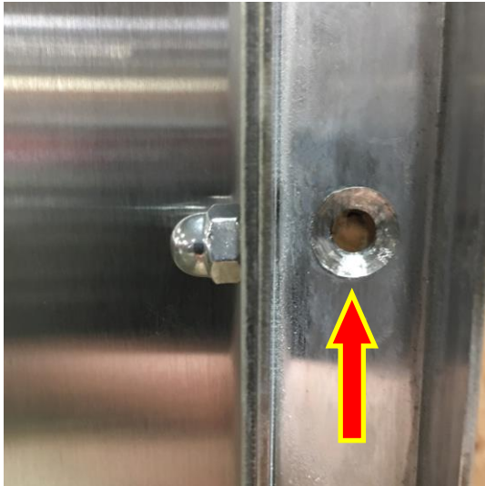
Figure 7: Predrilled holes within the door track for fastening the frame assembly to the wall stud
