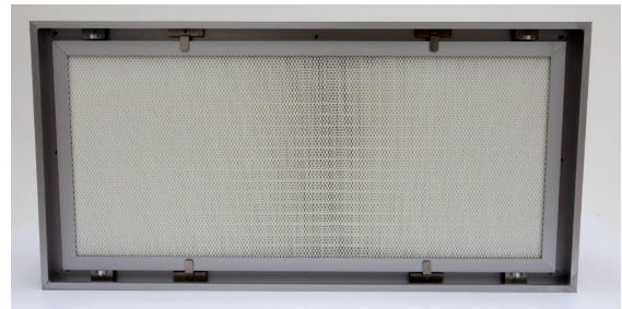
Figure 17: Exposed filter after removing protective screen
