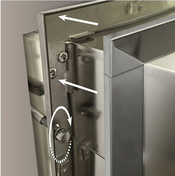
Figure 7: Thread the lag bolt into the guide attached to the “clean”-side bracket, sandwiching the wall between the brackets
